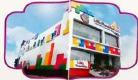
Kanpur Road Campus
